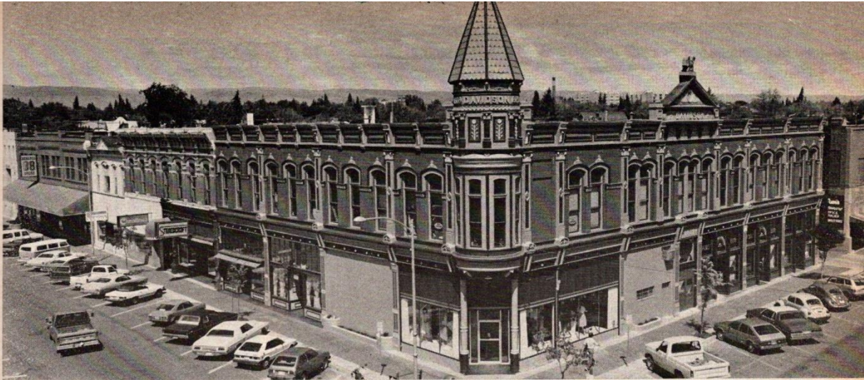
Its face primly painted, the impeccably-restored Davidson Building dominates corner of Fourth Avenue and Pearl Street
